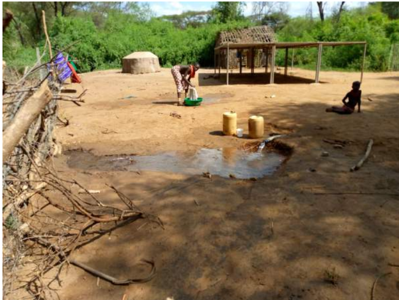
A massive hole where the standpipe was!
