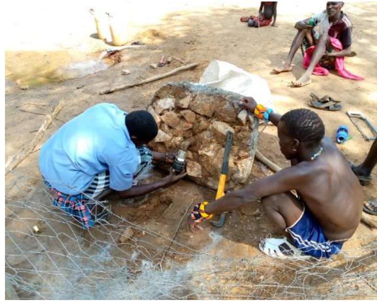
Building a more robust concrete plinth
